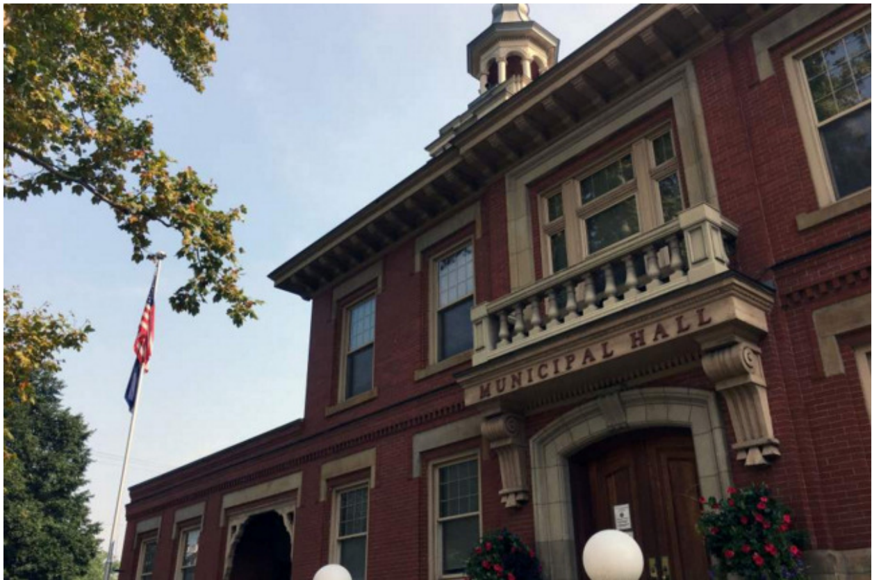
The Sewickley Borough Building.
